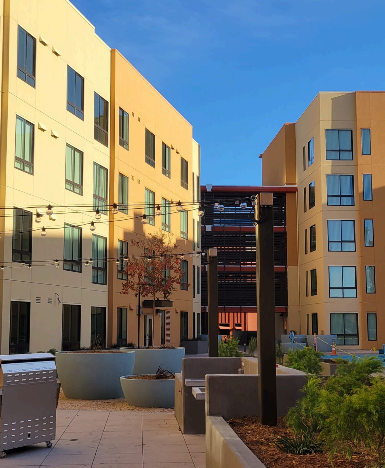
Casa Sueños, Fruitvale Transit Village Phase IIB, Oakland. 181 homes opened in January 2024.
